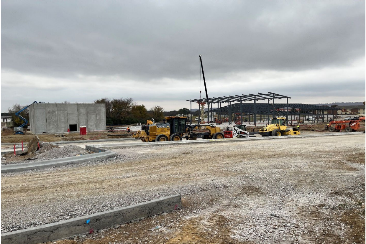
Figure 40 Sallisaw Child Development Center Construction
