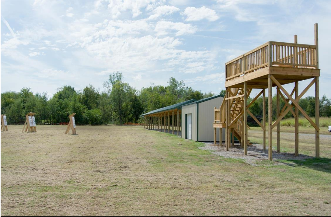
Shooting Barn and Platform (Reference Photo)
