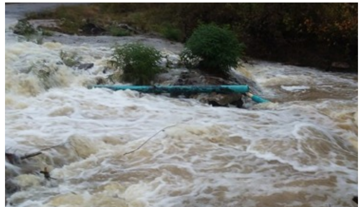
Washed out waterline – Oak Ridge, Adair Co, OK. Photo by Cherry Tree Rural Water District 10/24/19
