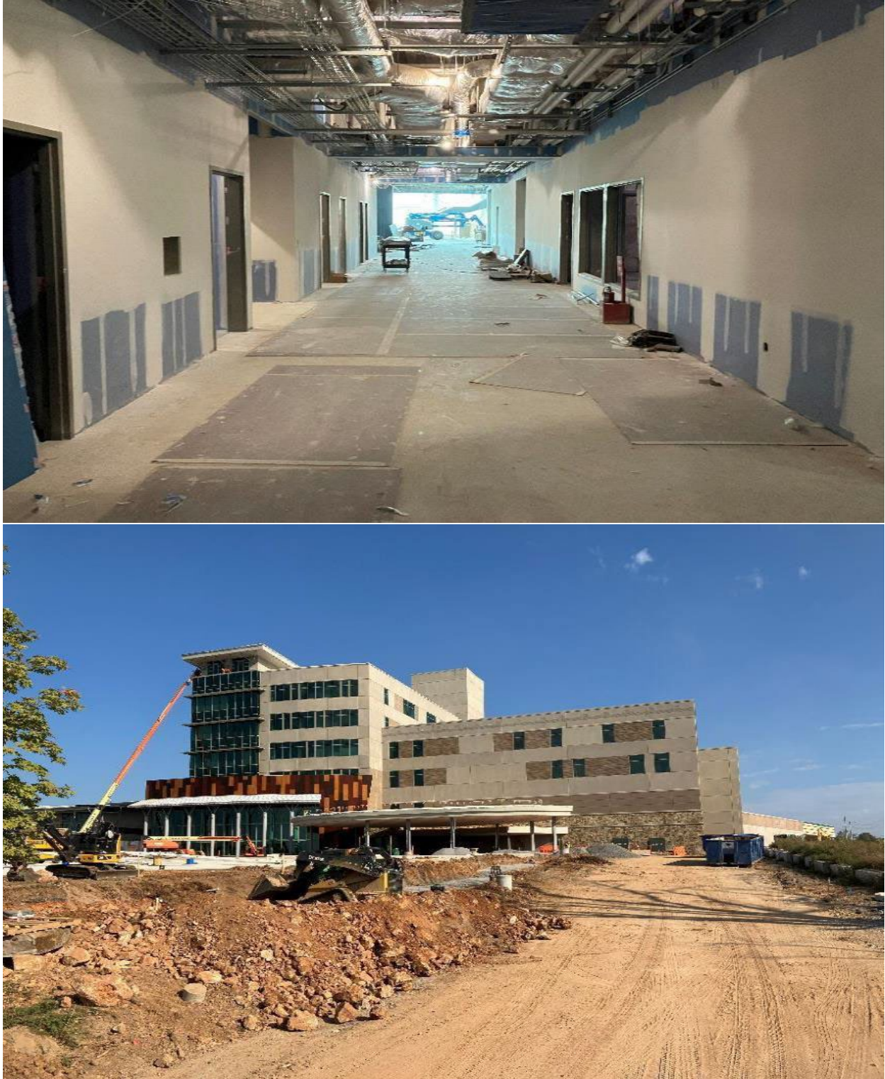
Figure 44 WW Hastings Hospital Construction
